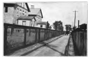
Fig. 79.—ALLEY IN EASTERN STEEL TOWN. COMMUNITY D. About 6½ feet wide, with 19-inch gravel walk on either side.
